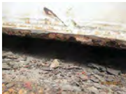
1. Bottom seal damage 2. Under floor plate corrosion
